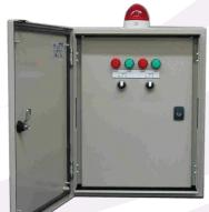
Standard level control system with inner door (float switch control)
